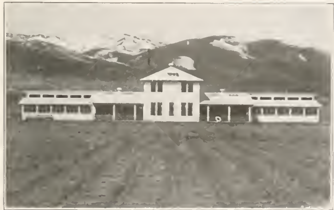
U. S. Indian Sanatorium at Carson, Nev., illustrating a standardized design much in use in hospitals of the Indian Bureau.
